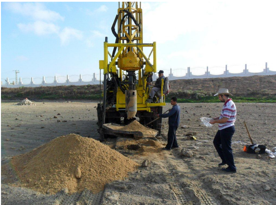
Figure (4-2): Drilling method using Rotary Auger
